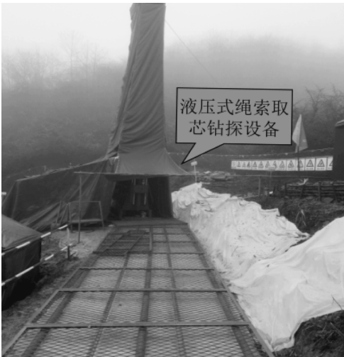
图 3 机台选用“架空式” Fig. 3 Overhead drilling crew
